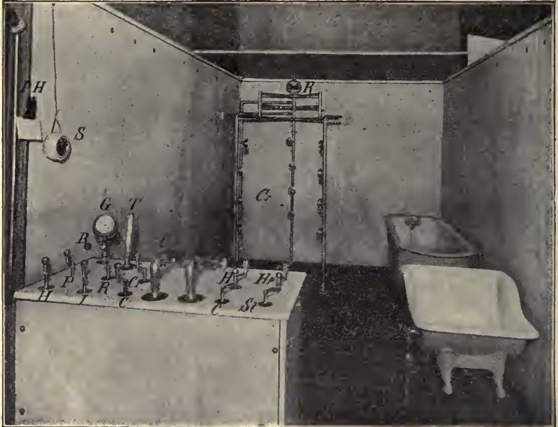
FIG. 48.—Baruch's Douche Apparatus. PH , Prescription-holder; S , "second" clock; H , hot water; I , ice water; C , cold water; P , pressure regulator; B , bell; G , gauge; T , thermometer; R , rain douche; Cr , circular douche; CJ , cold-jet douche; HJ , hot-jet douche; H , hot water for Scotch douche; C , cold water for Scotch douche; Hp , hip-bath; St , steam douche.
