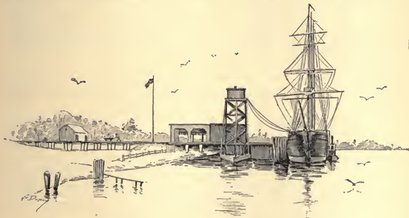
FIG. 61.—View of Disinfesting Wharf, showing Tug Fumigating Vessel; elevated tank containing eight thousand gallons of bichloride-of-mercury solution, three leads of hose from tank to ship. Gangway leading to building containing superheating chamber.
